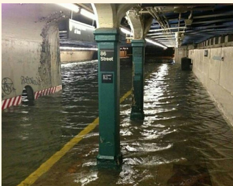
Figure 5.4. The nation’s busiest subway system sustained the worst damage in its 108 years of operation on October 29, 2012, as a result of Hurricane Sandy. Millions of people were left without service for at least one week after the storm, as the Metropolitan Transportation Authority rapidly worked to repair extensive flood damage (Photo credit: William Vantuono, Railway Age Magazine , 2012 46 ).
